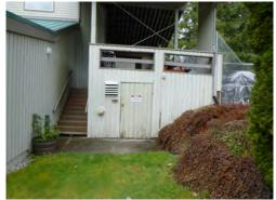
The clubhouse has several sections of deteriorating siding that will require replacement. Recommend inspection and repair of reported rot damage within the wall structure prior to replacement of the existing siding.
