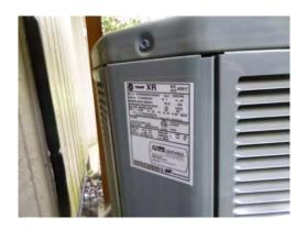
The clubhouse heating system was upgraded to a modern heat pump system in 2017. This type of equipment should provide a useful life of 15-18 years as it is not in full time usage. An allowance is also included for hot water heating equipment.
